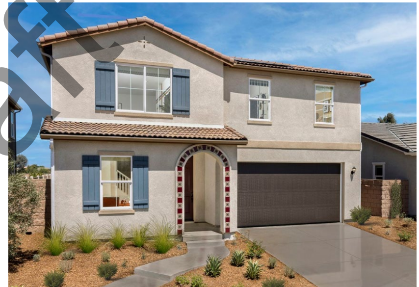
Similar Single Family Home 19180 El Gallo St. (Catania at Citrine), City of Riverside
