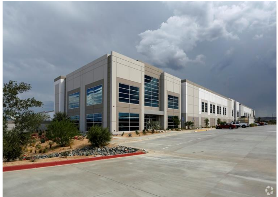
Example Prototype Industrial Development, City of Perris
