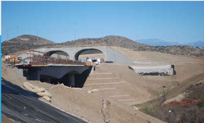
The wildlife crossing, pictured above during project construction, provides a safe way for wildlife to access habitat on both sides of the new roadway. The bridge over Warm Springs Creek is also pictured.
