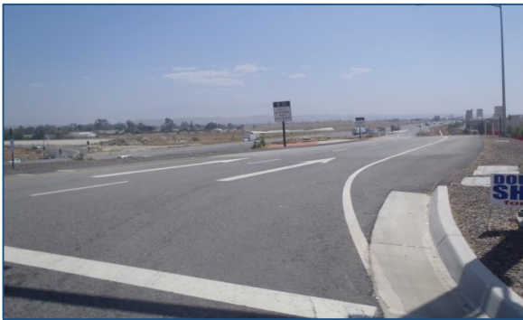
Eastbound On-ramp from Nason Street
