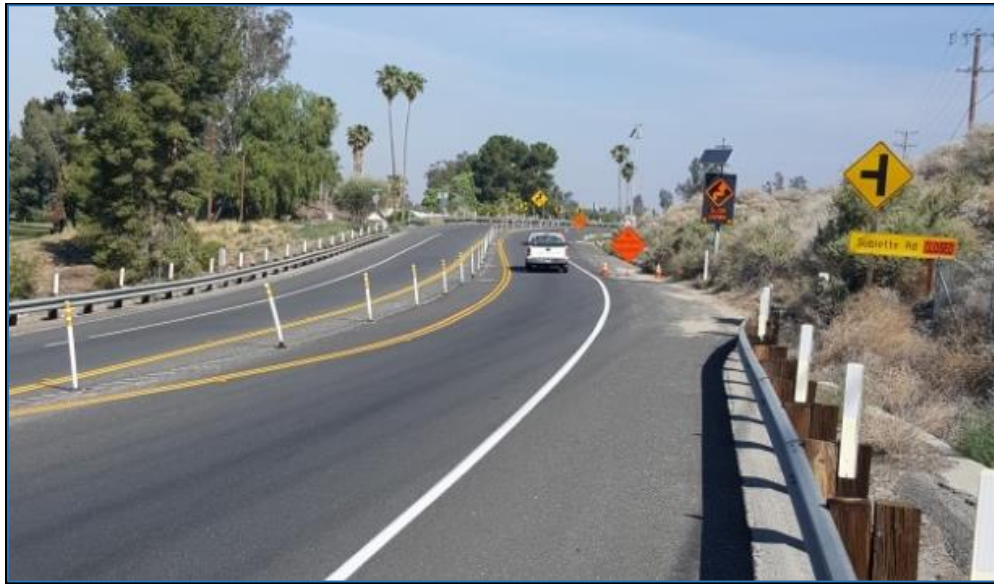
Section A – Gilman Springs Road (State Street Boulevard to Country Club Drive) Facing Northbound
