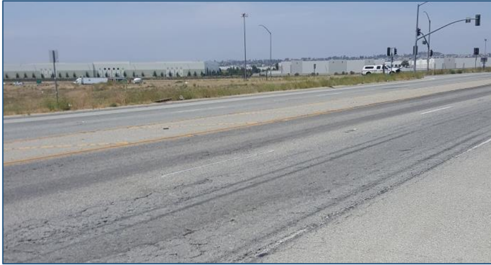
Section D – Cactus Avenue (Elsworth Street to I-215) Facing Westbound
