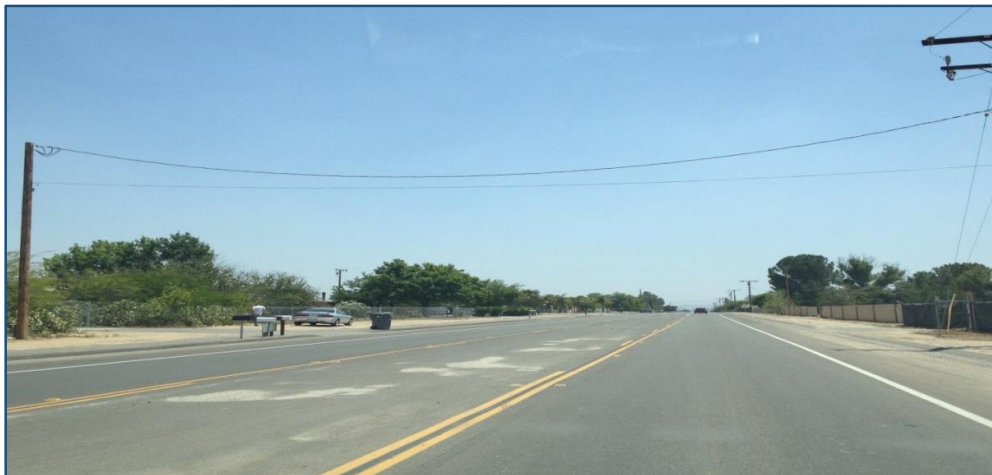
Section C – Evans Road (Orange Avenue to Water Avenue) Facing Northbound
