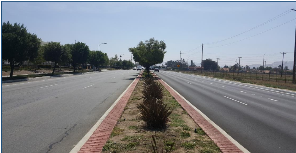
Section A – Cactus Avenue (Heacock Street to Gilbert Street) Facing Northbound
