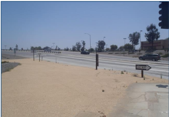
Eastbound Off-ramp onto Day Street
