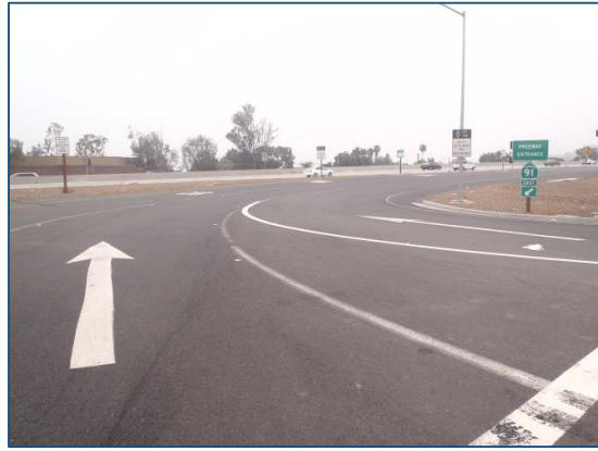
Northbound On-ramp from Indiana Avenue
