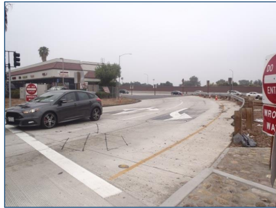
Northbound Off-ramp onto Indiana Avenue
