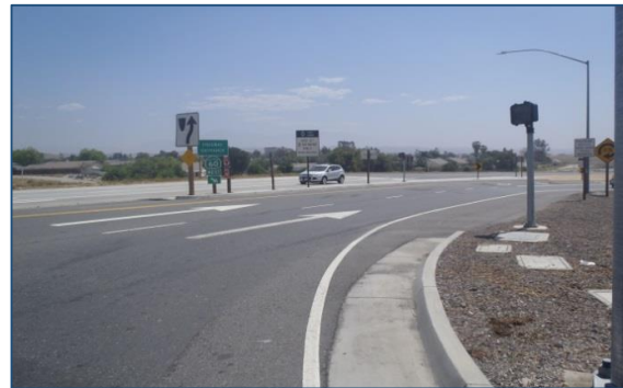
Westbound On-ramp from Nason Street
