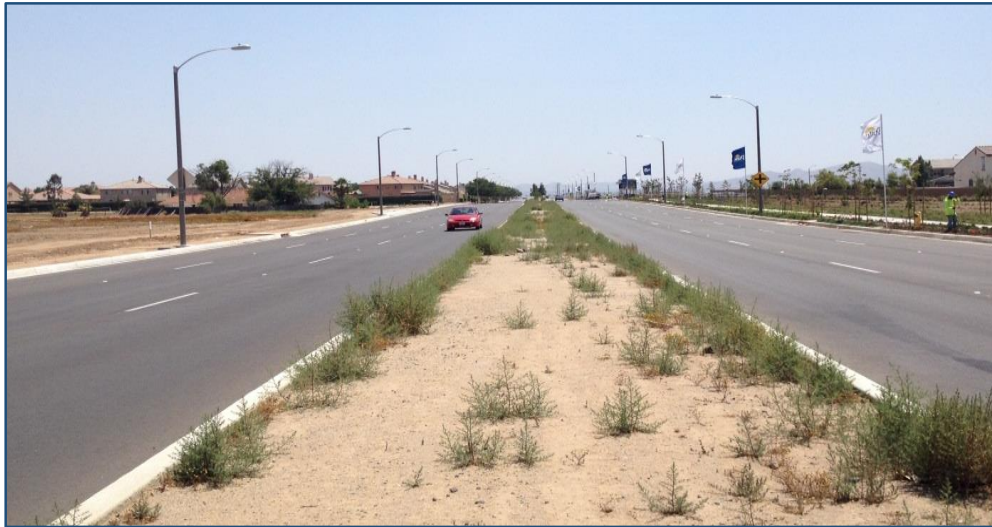
Section D – Evans Road (Water Avenue to Placentia Avenue) Facing Southbound
