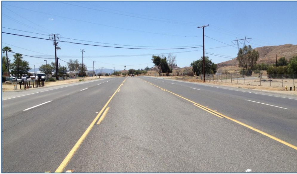
Section A – SR-74 (Ethanac Road to Trellis Lane) Facing Eastbound
