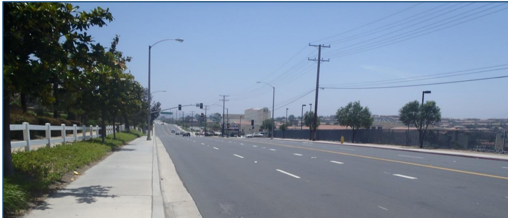
Section A - Wood Road (Bergamont Drive to Martin Luther King High School) Facing Southbound
