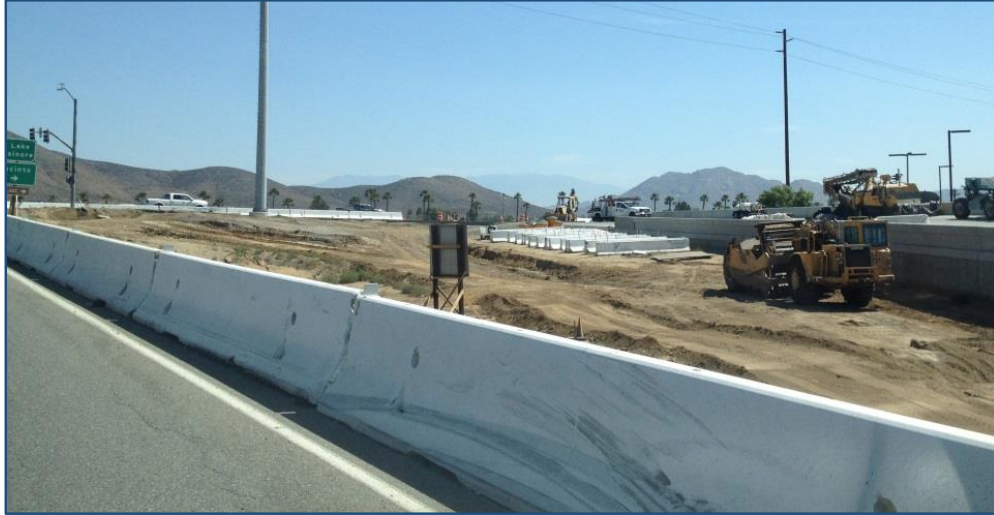
Newport Road/I-215 Interchange Southbound Off-ramp
