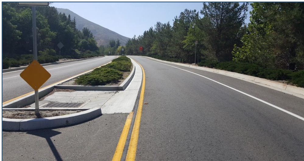
Section C – Gilman Springs (Golden Era Productions to Sanderson Avenue) Facing Eastbound
