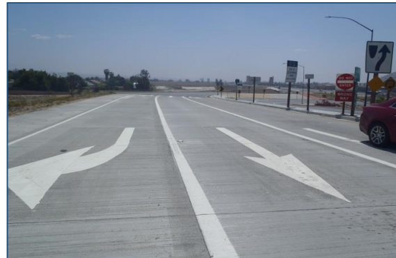
Westbound Off-ramp onto Nason Street
