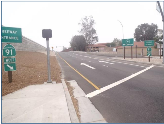
Southbound On-ramp from Arlington Avenue
