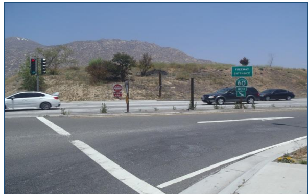
Westbound Off-ramp onto Day Street
