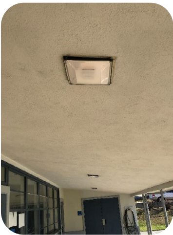
Above: Lincoln Elementary School
