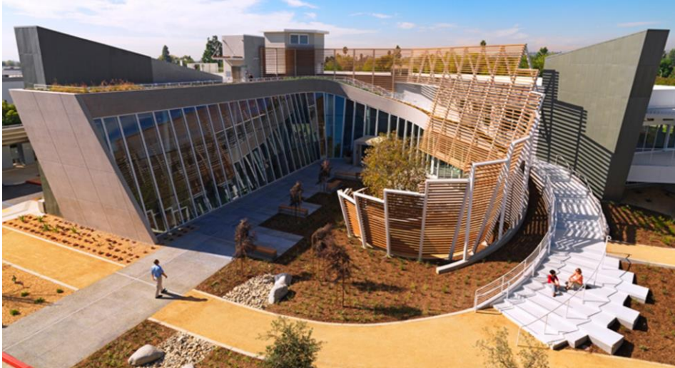
The Frontier Project, Rancho Cucamonga – Demonstration of water and energy conservation
