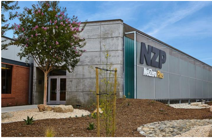
Net Zero Plus Electrical Training Institute, Los Angeles – High Tech Building demonstrations and training
