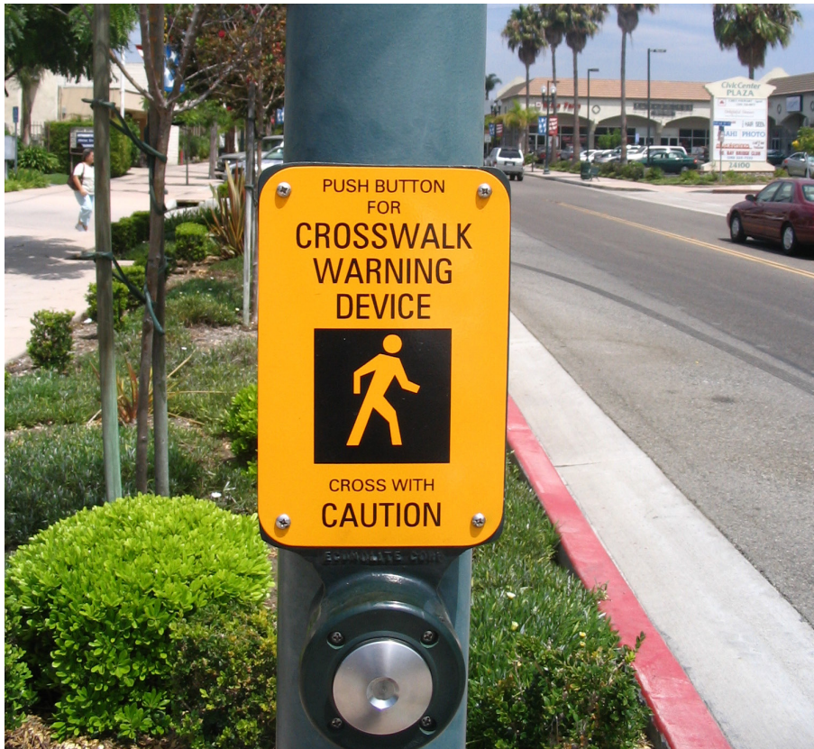
Crosswalk pushbutton for pedestrian warning device
