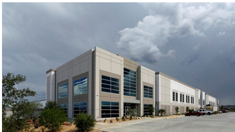
Example Prototype Industrial Development, City of Perris
